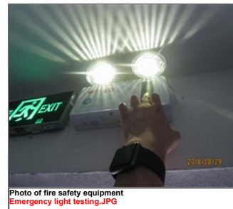
Photo of fire safety equipment Emergency light and directional sign in the staircase.JPG
